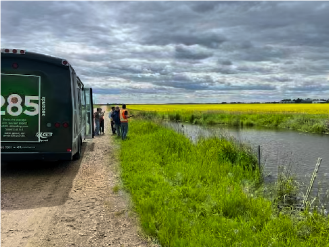
Looking at sink hole.
